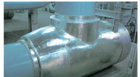
Finished article (spraying insulation)
