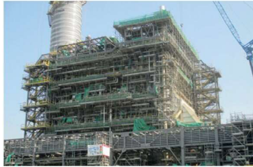
Construction site in Hong Kong (CLP Power D-Station)
