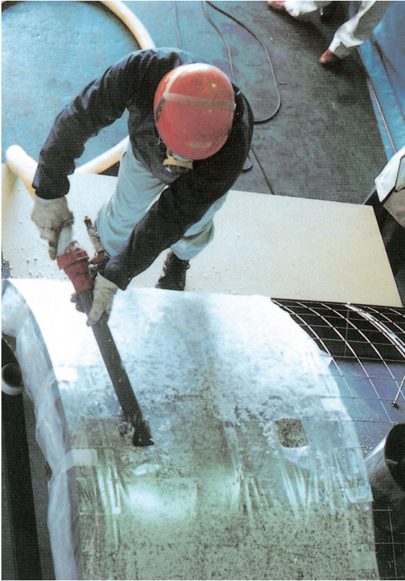
To spray the insulating material
